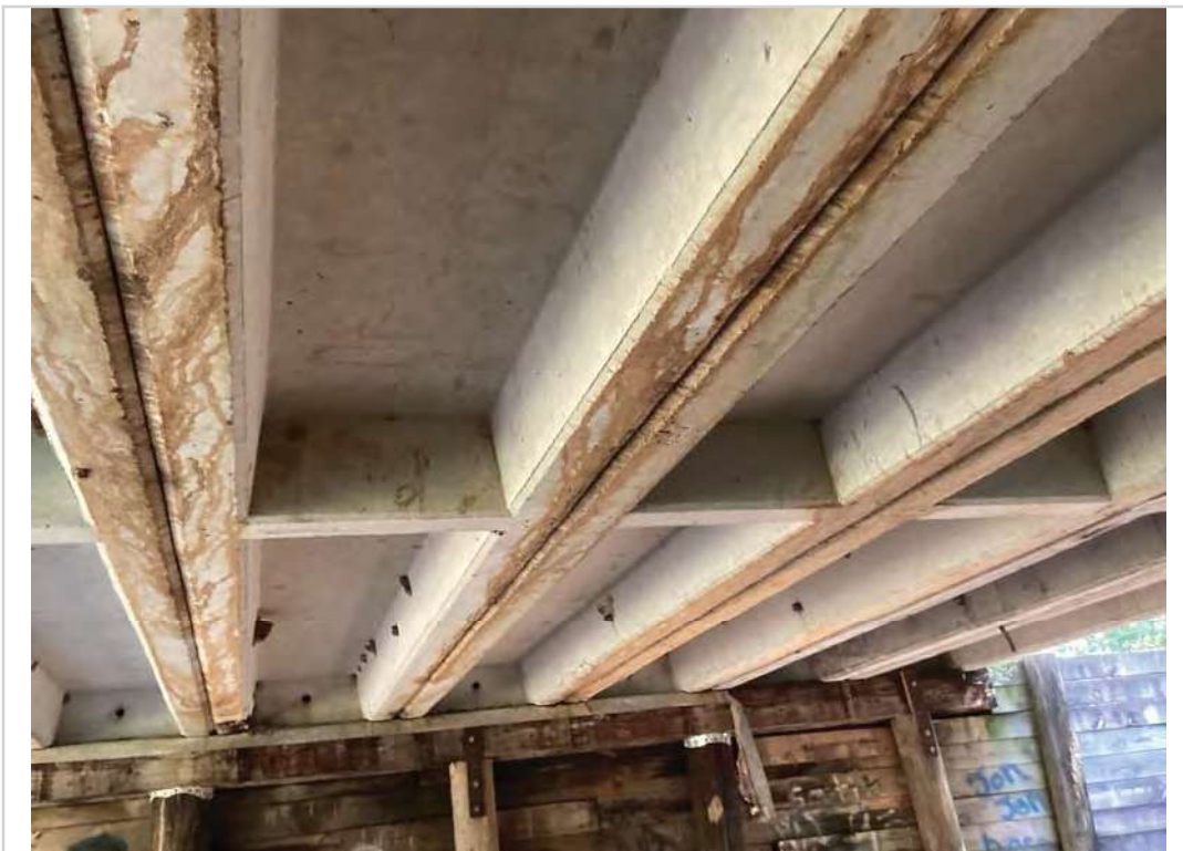
Bottom deck span 1 typical
